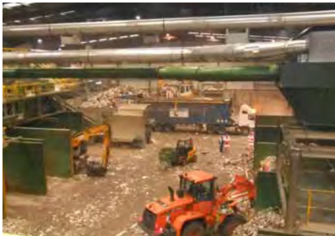
Materials recovery facility
